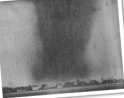
The tornado approaching Moore Lake
